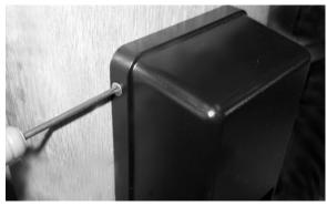
FIG. 16: SECURE TOP OF INSIDE HOUSING
